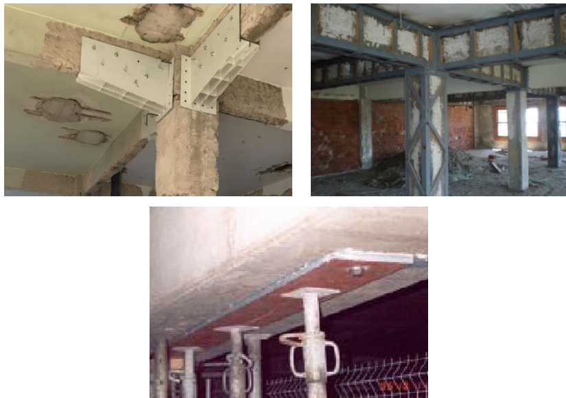
Figure 2. Strengthening with steel profil0065
