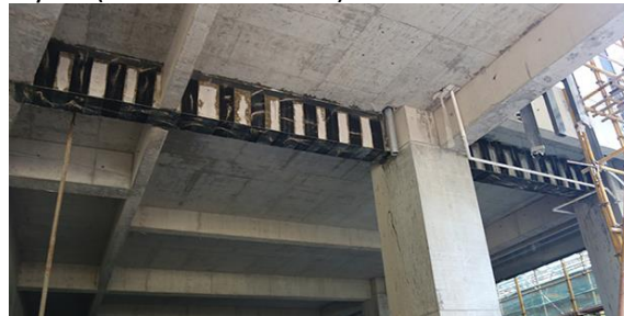
Figure 1. Strengthening with FRP
