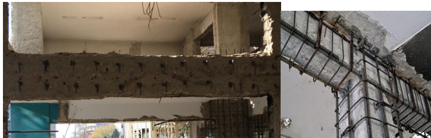
Figure 3. Strengthening with Jacketing or External Stirrups (Seckinli, 2018) and www.imagenesmy.com
