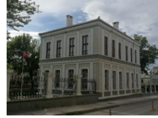
Figure 6. Second mansion in the area of governor's office, 2020
