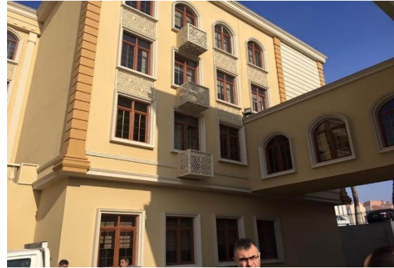
Figure 8. Government house after renovation (Raymimarlık, 2021)
