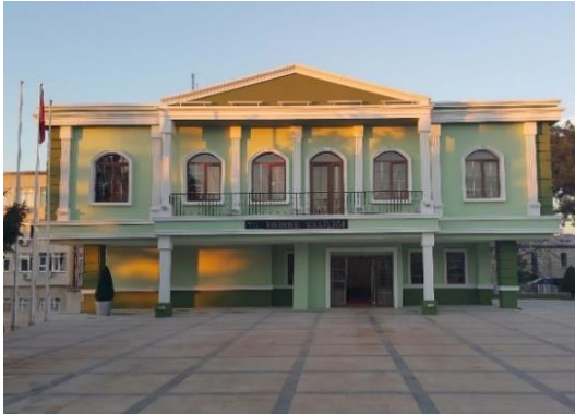
Figure 7. Governorate entrance after renovation (Visitturkey, 2020)
