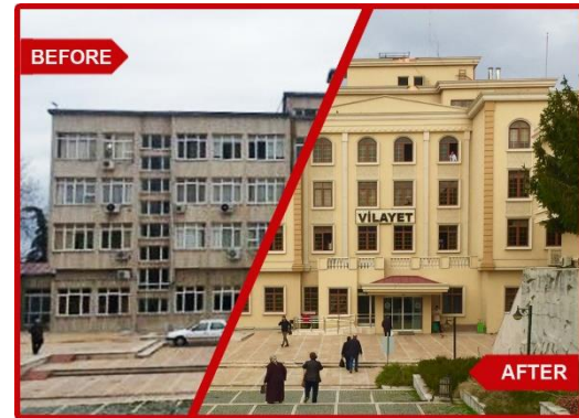
Figure 10. Before and after of the main Government House 4
