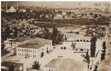
Figure 1. Buildings in Paşakapısı in the last quarter of the 19th century (Edirne, 2020)
