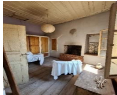
Figure 4 First floor pic 2
