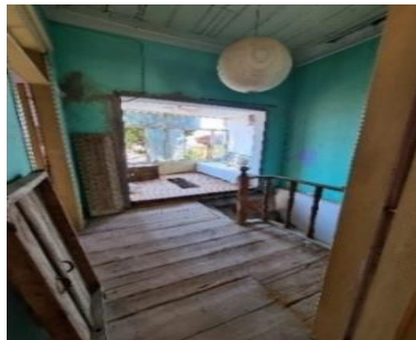
Figure 3 First floor pic 1
