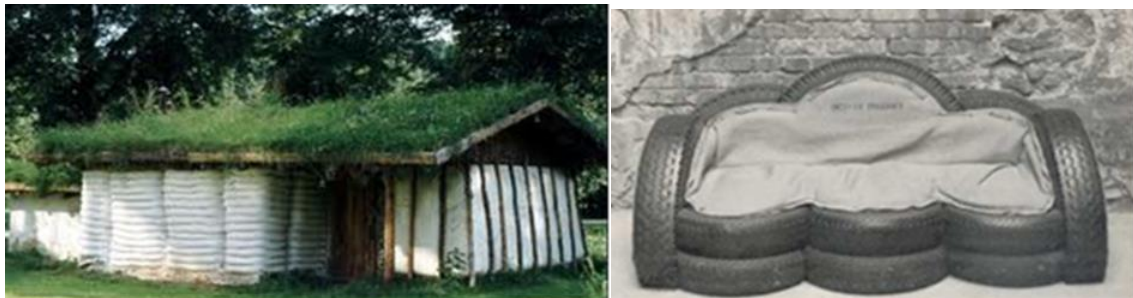
Figure 1: Sandbag and textile shelter realized by Gernot Minke in Guatemala ( www.gernotminke.de/ )
