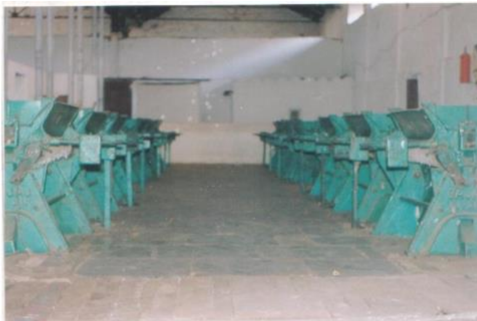
BATTERY OF DOUBLE ROLLER (DR) GINNING MACHINES
