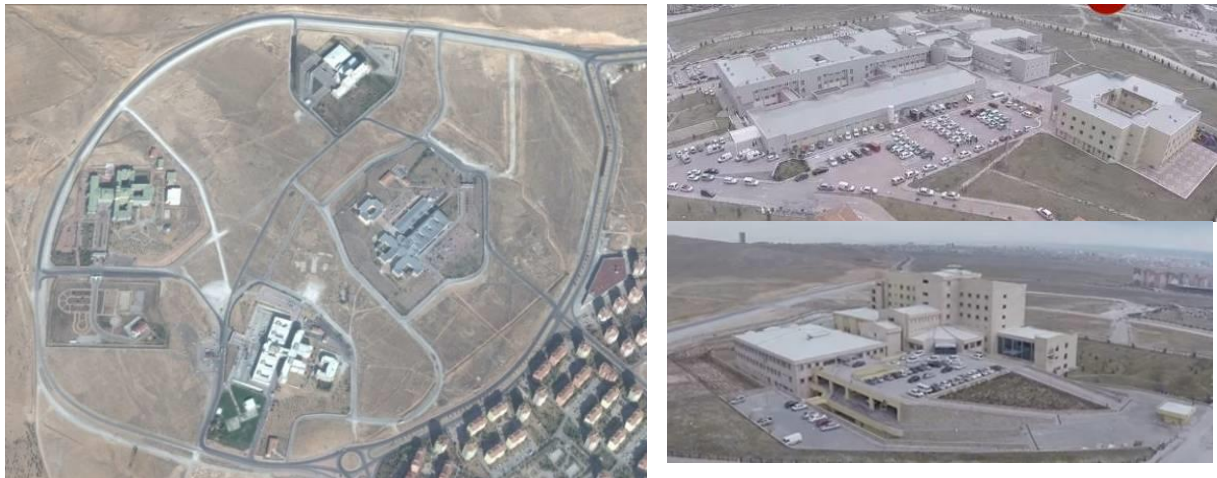
Figure 13. Hospital zone and general view of hospitals
