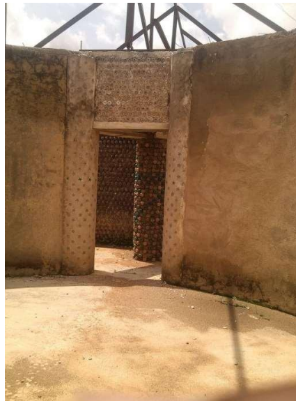
Figure 8. Generic plastic bottle used to construct the structural elements of this building
