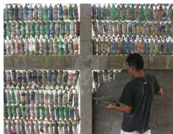
Figure 2. Column and beam in plastic bottle masonry construction
