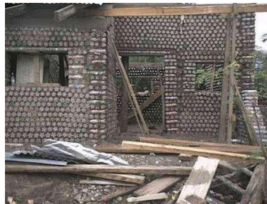
Figure 4. Square column using reinforced plastic bottles Source: The houses that PET plastic built – Recycle bank.
