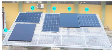
Figure 2. PV modules installed
